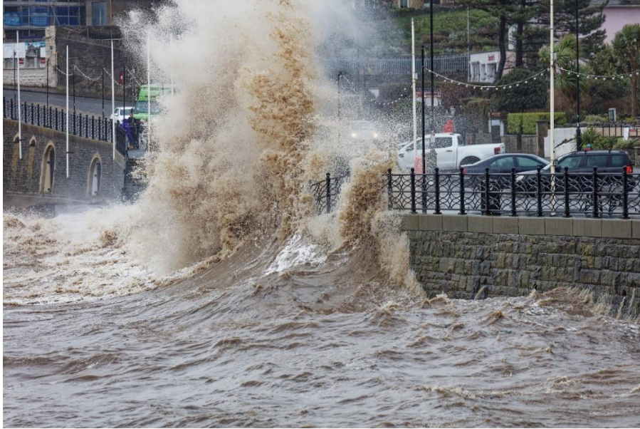
Images 1 and 2. The Victorian sea walls at Clevedon protect residents from flooding when there is a combination of high tides and stormy weather.
